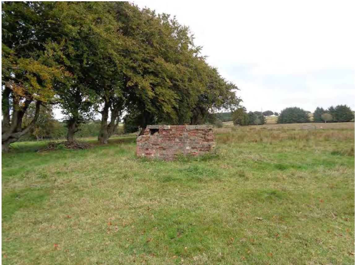
Plate 20: Small modern brick structure at northern end of study site
