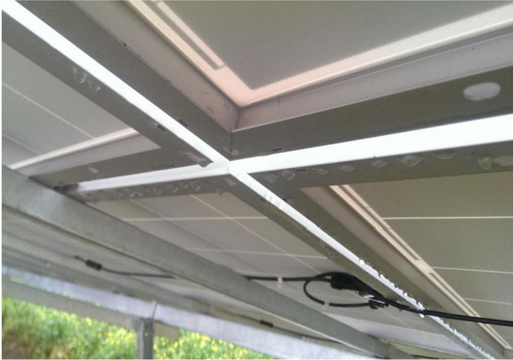
Figure 10. Underside of a solar panel
