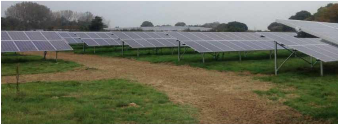
Inserts 10 and 11: Localised Repairs (solar farm in Sussex)
