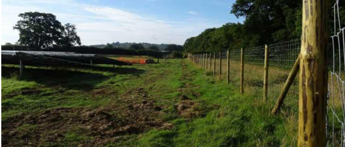
(The photos in this section were taken on heavy, clay soils with poorly draining subsoil, and the work was photographed in July and August 2015)
