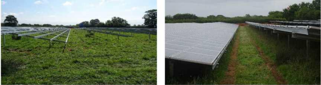
Inserts 29 and 30: Ground After Construction (example from Wiltshire)
