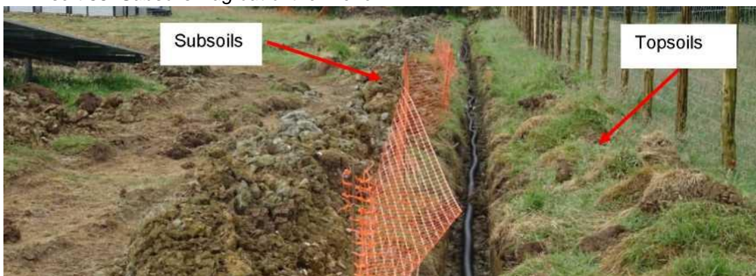
Insert 38: Subsoils Dug out of the Trench
