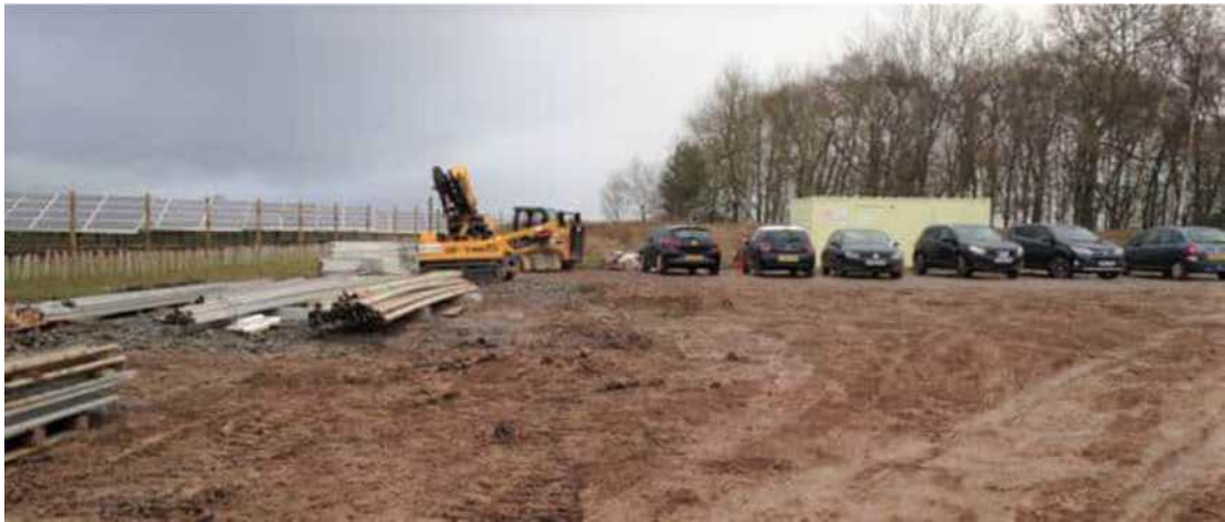
Insert 17: Start of Restoration of Construction Compound (example from Staffordshire)
